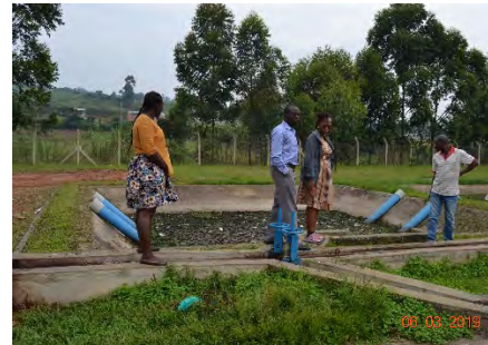
Team at the Sewerage treatment area
