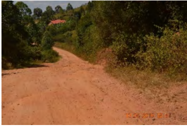
Road at Municipal boundary East Ward
