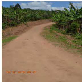
Access road to Ahakatogo centre
