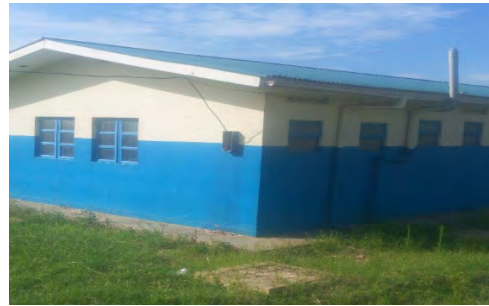
National Water and Sewerage Corporation, Offices, Ntungamo
