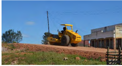
Road near Eastern Ward Offices, under construction
