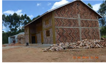
Factories along Mbarara – Kabale road
