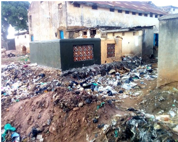
Plate 33: Typical Garbage Bunker
