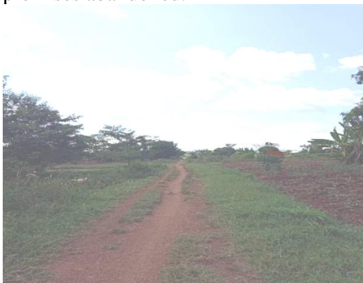
Plate 27: Dysfunctional rail route where Road rails were vandalised
