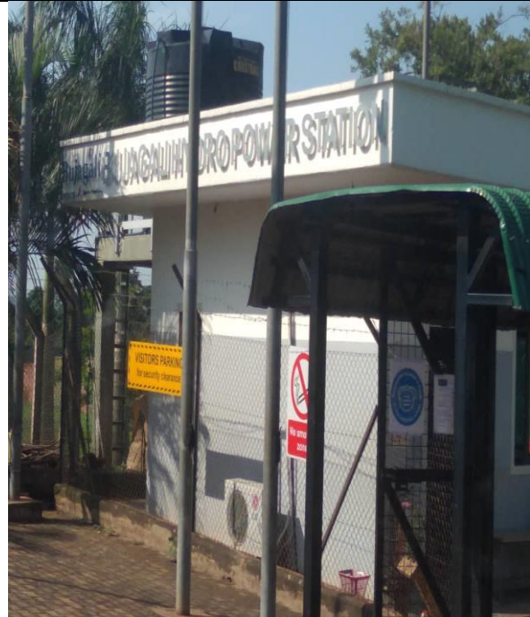
Bujagali power station
